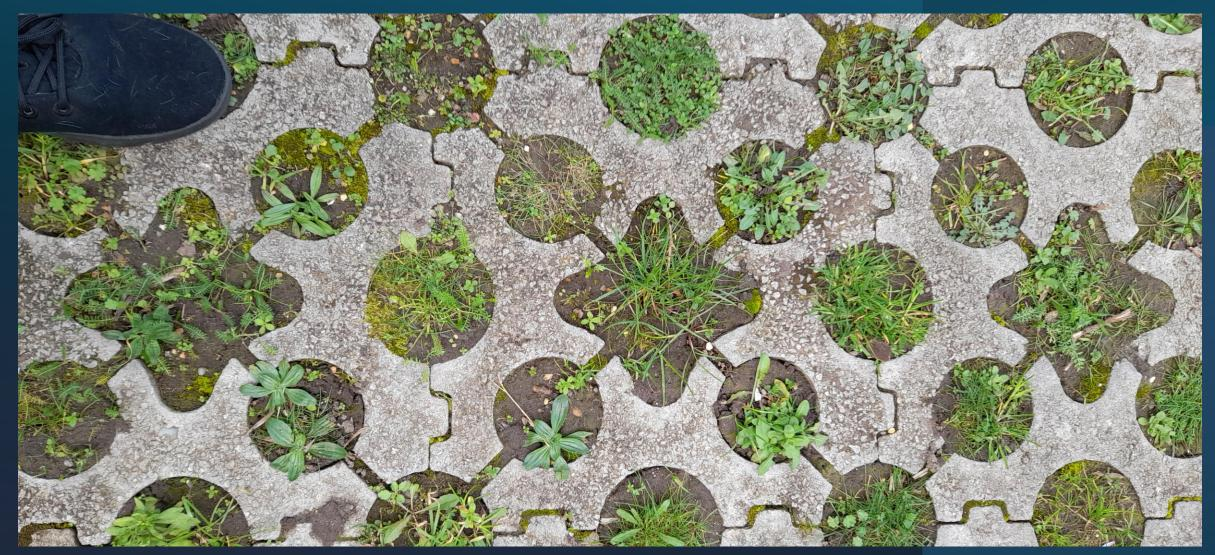
**Matrix paving** takes vehicles but without the 'need' to remove soil, is truly permeable, rather than the kinds of **"permeable paving"** being marketed (which is precast concrete, made to look like stone or brick), and can be planted up with different species to keep 'weeds' from dominating.
